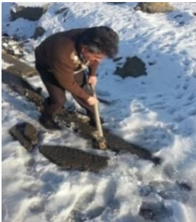
Fig 1. Asphalt samples prepared by removing road surface
